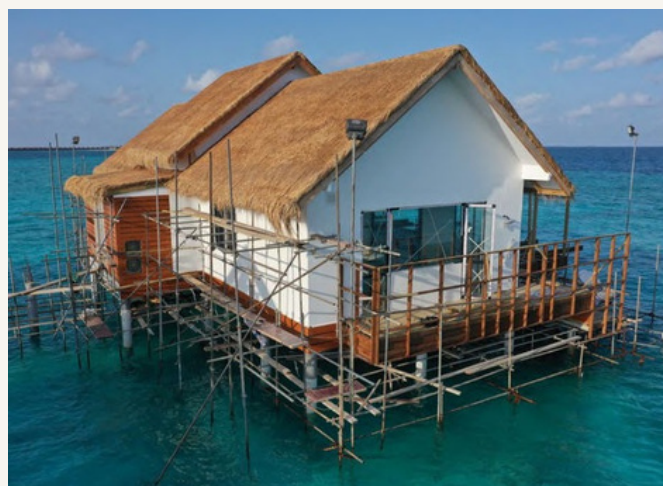
Completed external cladding example.
