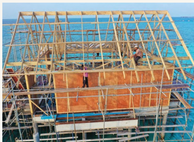
Panels installed on a coastal project.
