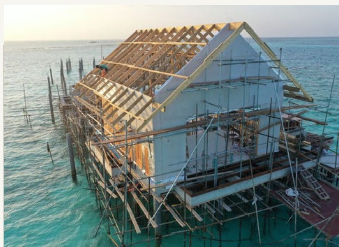
Pre-manufactured panels beneath the exterior finish.
